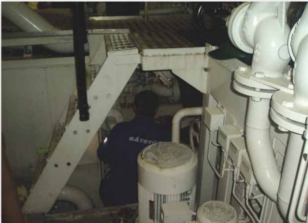
Appendix 8.4.1 Photograph of general area of port valve chest
