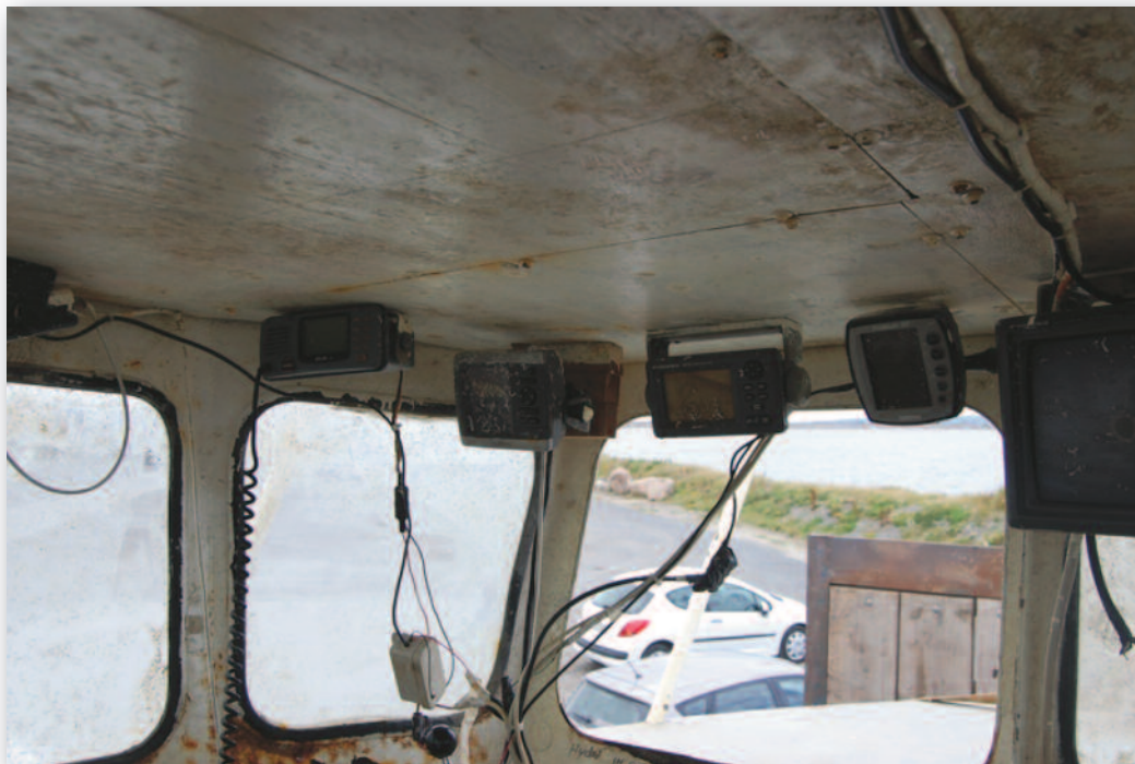
Photograph No. 5 - Showing wheelhouse with missing window
