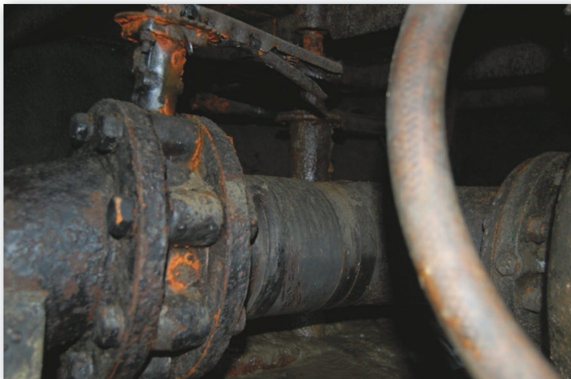
Photograph No. 6 - Showing Dredging cage water pump
