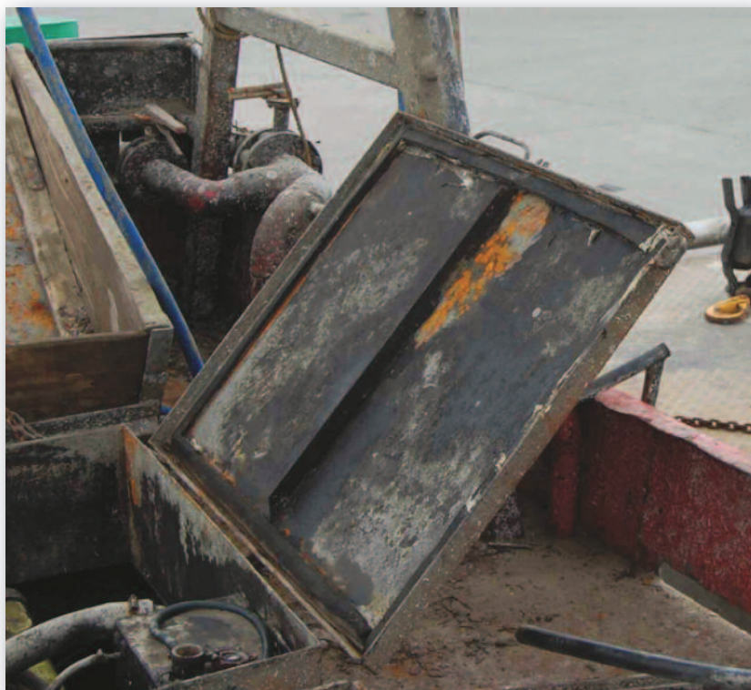
Photograph No. 4 - Showing hatch cover
