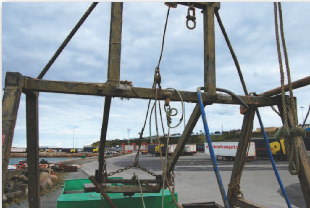
Photograph No. 7 - Showing Gantry
